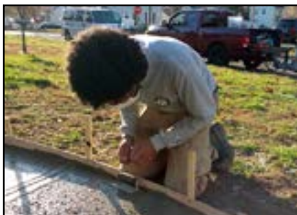
River 4's Tree Moses separates the concrete from the form so when the form is removed, the walkway isn't damaged.
