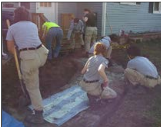
The River 4 team guided by Greater Springfield Habitat for Humanity (GSHFH) Construction Manager Sheri Green, in the neon green shirt, levels the surface of the old walkway for the new path and clears away dirt from the edges to make room for the form.
