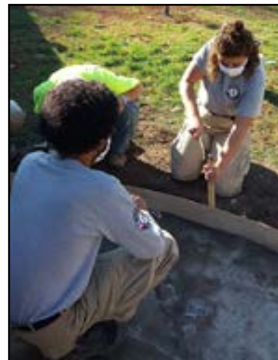
River 4's Milynn Scott hammers in a stake to secure the form for the new pathway. Her teammate Tree Moses watches.
